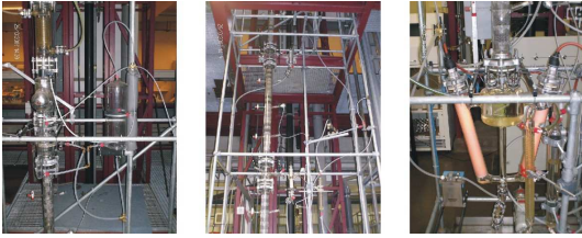
Fig. 2. Pictures of the pilot-scale distillation column: condenser (left), packed section and feed introduction (center), and reboiler (right).
