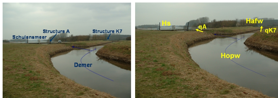
Fig. 5 Photo of the river Demer and the "Schulensmeer" flood control reservoir in the background, together with the locations of the main water level and discharge variables.
